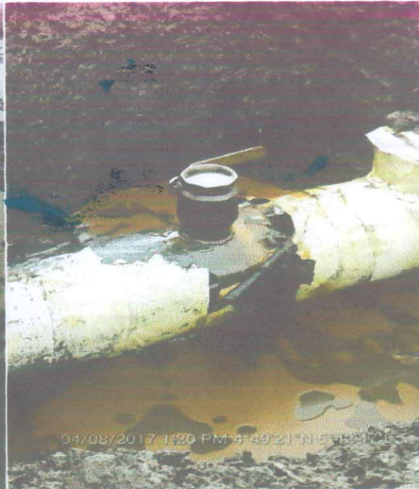
3" Valve installed by vandals
