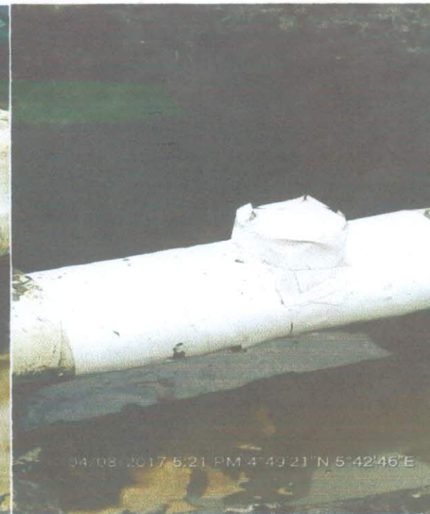
3" Valve installed by vandals
